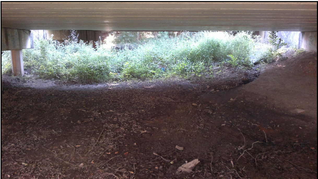
Albany Creek Road – Looking Downstream
